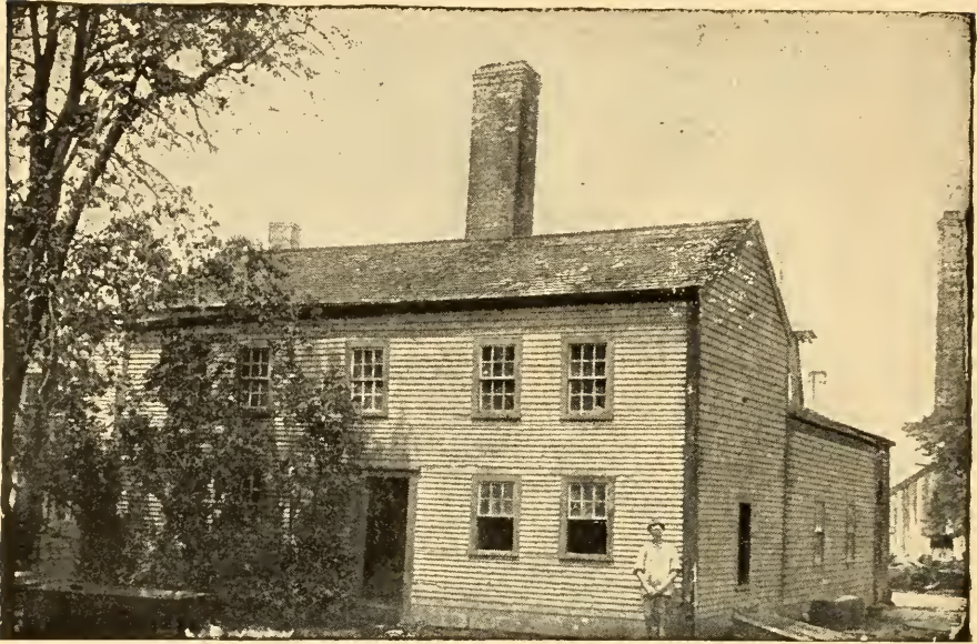
Revere House at Canton.
